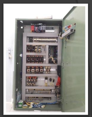
Panel controller with PLC and/or embedded PCB for any machinery purposes
